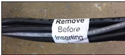
Uncoil the bundle of pre-wired cables from gantry and remove temporary cable wraps.
