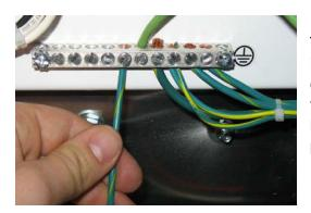
Take bare end of the green ground wire, and connect it to any available spot on the ground bus. Loosen one of the screws until the wire slips into the gap, and tighten screw.
