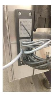
**LEFT:** For an lcotec cord fixture, remove the 3 bolts from the left side of the black fixture, and pull the side out. Remove one of the bottom gray squares, and run accessory cable into the control box, using one of the plugged holes in the gray square cable holder. Slide the gray square back in place, and reattach the left side to the fixture, making sure the cable reaches the driver.
