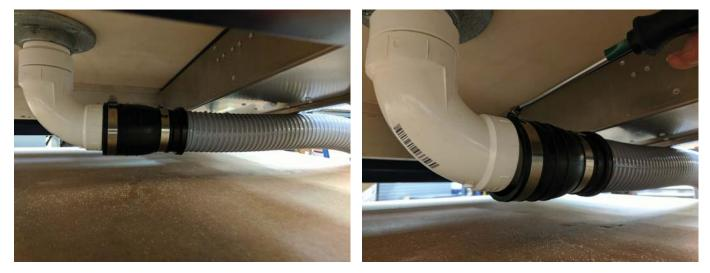
Make sure the hose is routed under the cutout section of the frame, and then lower the machine down carefully. make sure there is enough clearance under the machine for the hose. If the hose is being crushed by the machine, raise the leg levelers a bit more.
