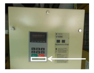
There are two main types of VFDs, a 10" model and a 16" model. These can be easily differentiated by their size and model numbers. Model numbers are found on the front of the VFD underneath the "RUN" and "STOP" buttons as shown to the left.
