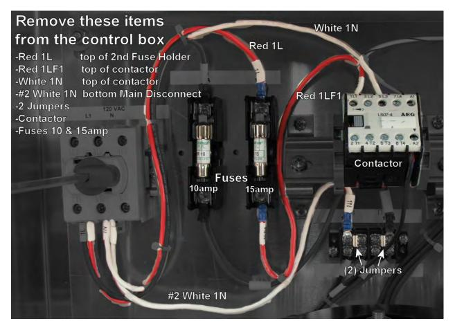
Trace the last two wires connected to the existing contactor and remove them from the control box all together. (**Red 1LF1**) will be removed from the bottom of the 2nd fuse holder. (**White 1N**) will be removed from the bottom of the main disconnect 4T2. While there, remove the (**#2 White 1N**) from the same main disconnect location. The other end is on small terminal connection under where the contactor was located.
