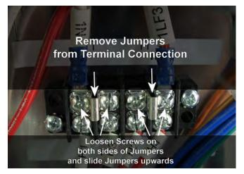
To finish out all that is needed to be removed, remove the (2) jumpers located on this terminal. Loosen the screws on each side of the jumper and slide the jumper toward the top of the control box to remove.
