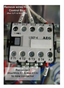
Remove the contactor wires from the existing contactor starting with **position A1** (Blue/White K1-) and **position A2 (Blue K1+A)**. These will be reconnected later into the new contactor, let them hang for now.
