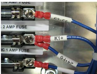
Loosen the right side of the 24V DC 2 amp fuse connection (middle glass fuse) and secure the new forked connection for (K1+)with the existing wire marked (24+F6).
