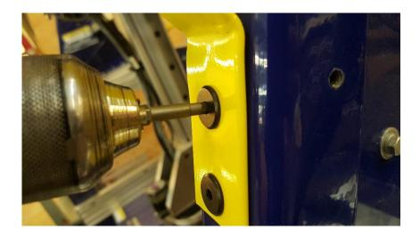
To make installation easier, use a drill or cordless screwdriver to torque down each bolt. Use a deep socket with drive extension to reach the nuts inside the gantry.
