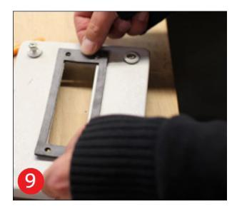
Tape the gasket around the wall cut-out
