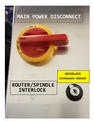
After the electrician has hooked up the PRSstandard control box, open the side of the box with a screwdriver (quarter turn locks). For safety reasons, the door is designed to lock open or closed unless the main power disconnect is turned off.
