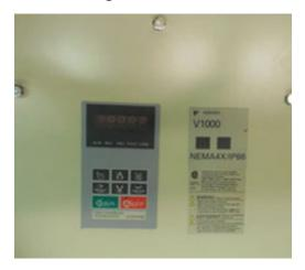
There are two main types of VFDs, a 10" model and a 16" model. These can be easily differentiated by their size and model numbers. Model numbers are found on the front of the VFD underneath the "RUN" and "STOP" buttons as shown on left.
